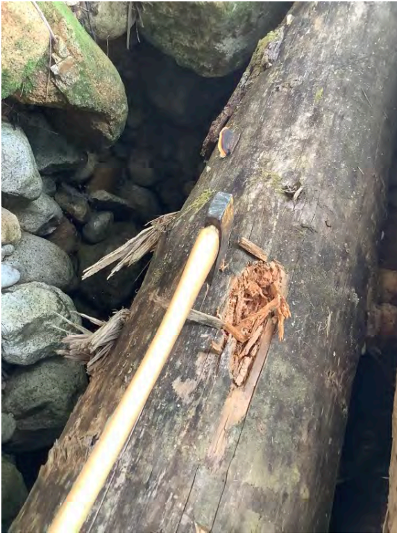
Stringers - upstream side
